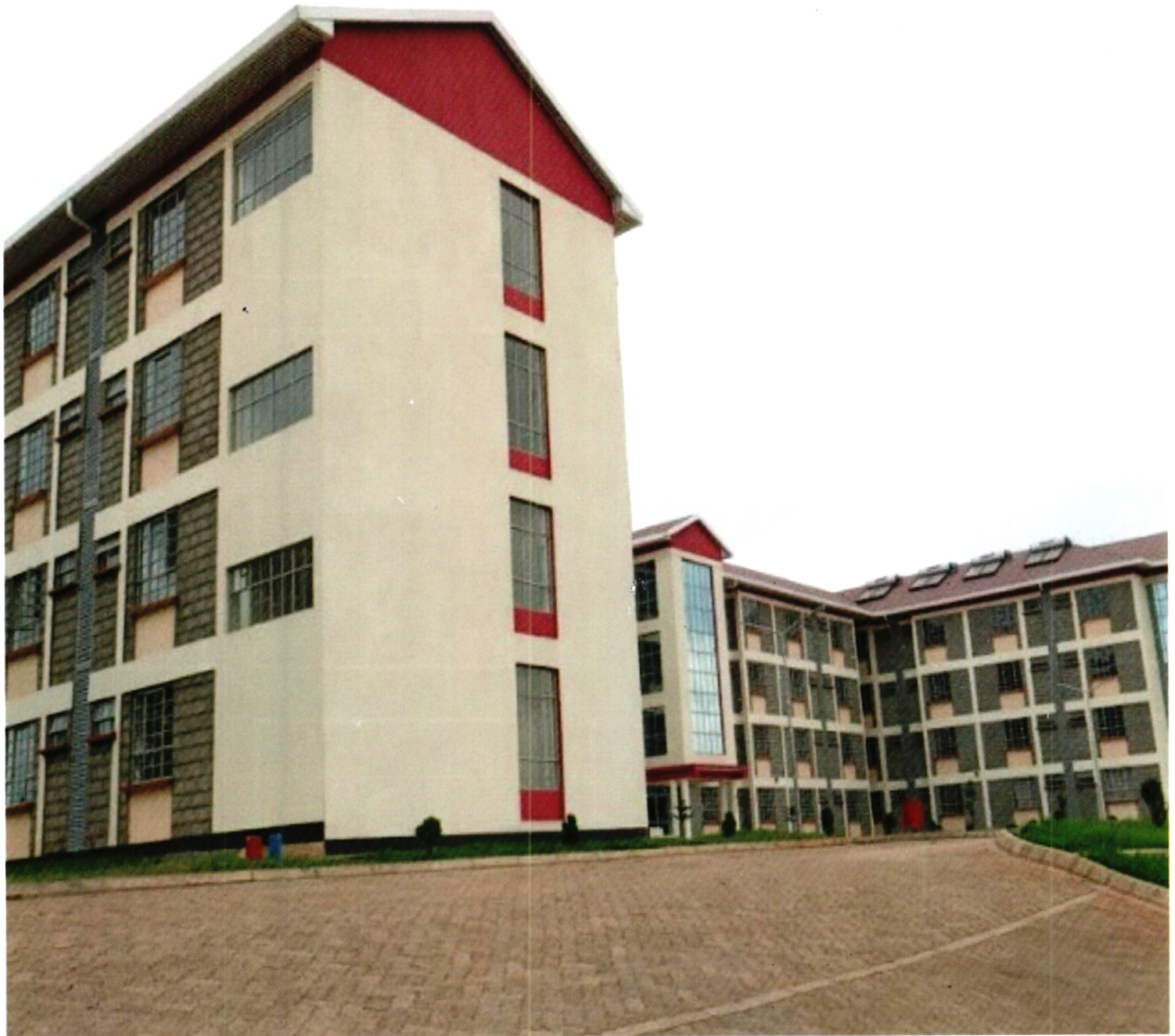
WOs' & SGTs' Single Accommodation at Moi Air Base
