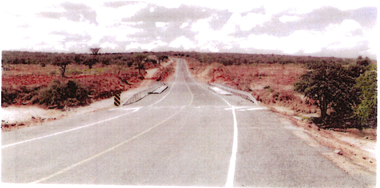
Completed Bridge in Kajiado – Imaroro at Km 32+298
