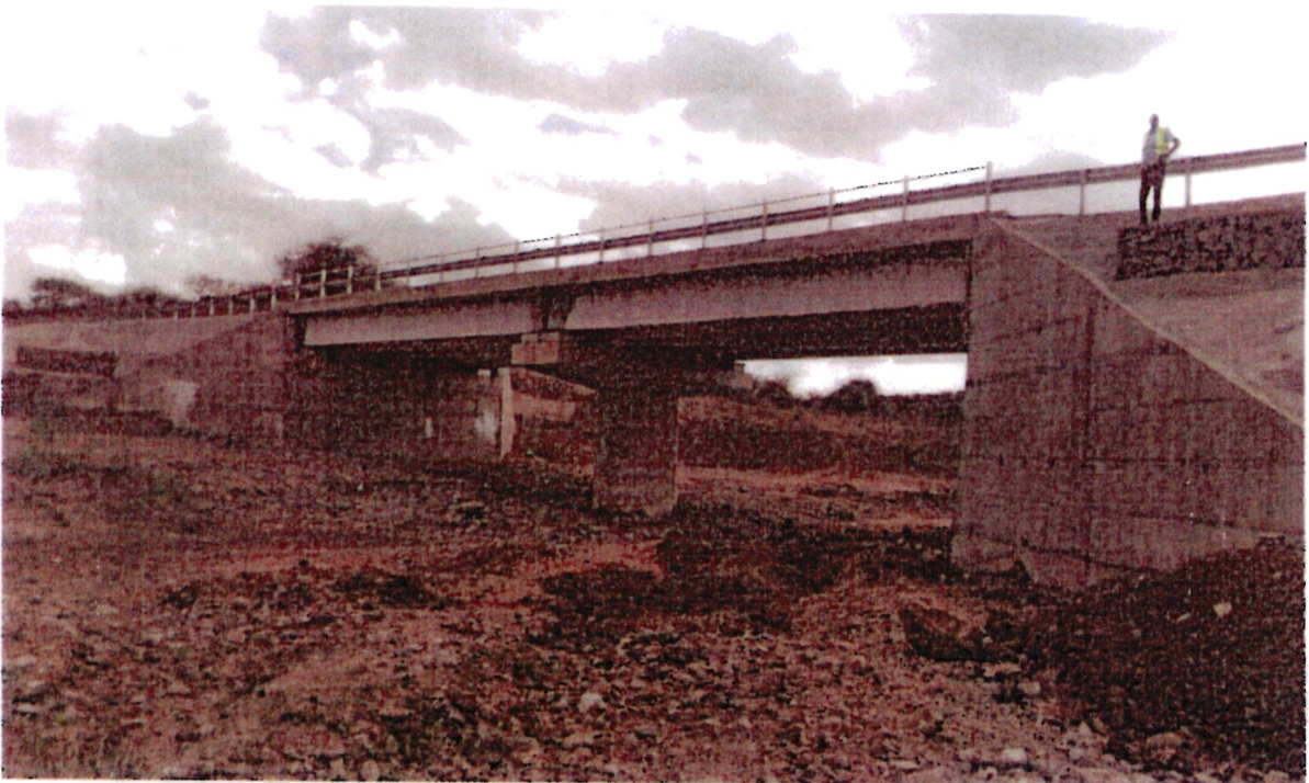
New 32m long two span concrete bridge at KM 32+777 along Kajiado – Imaroro project corridor
