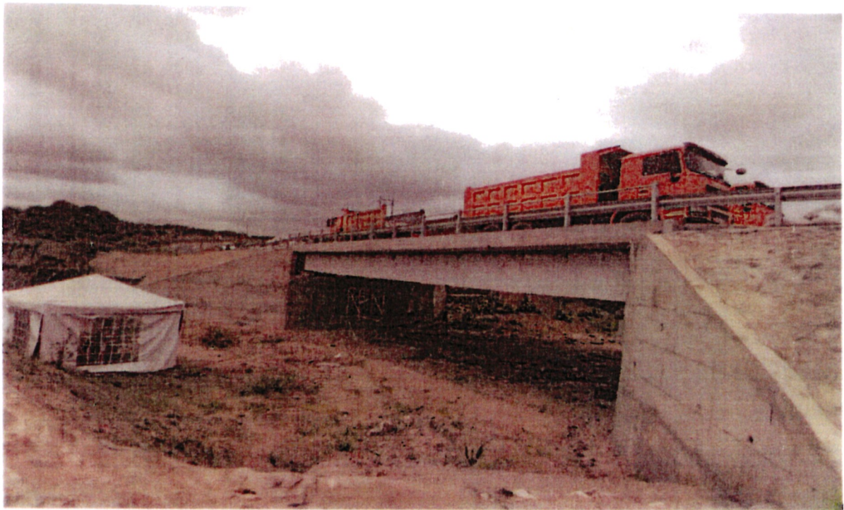
New 20m long single span concrete bridge at KM 17+757 along Kiserian – Isinya project Corridor
