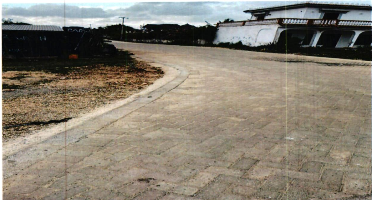
Cabro paving of Blue Jay to Kongo Mosque road
