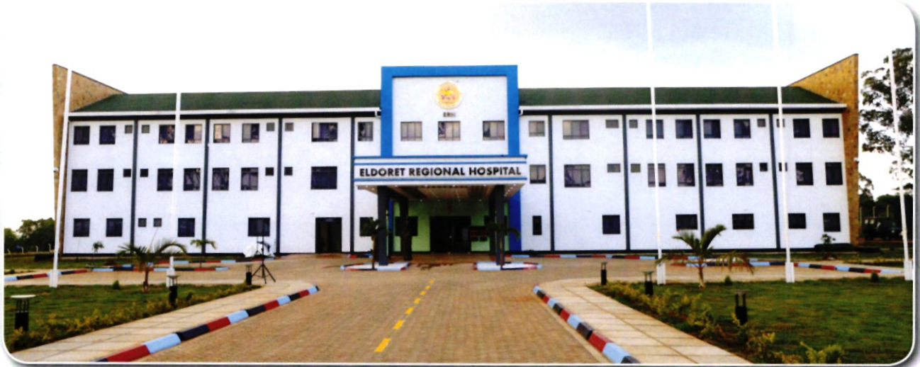
Front view of the completed Eldoret Regional Hospital (ERH) at Moi Barracks as at 30 June 2022
