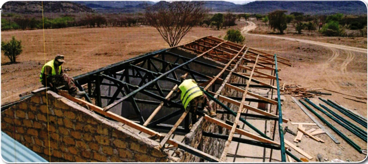
Renovation of Kapedo Mixed Sec School by the KDF soldiers
