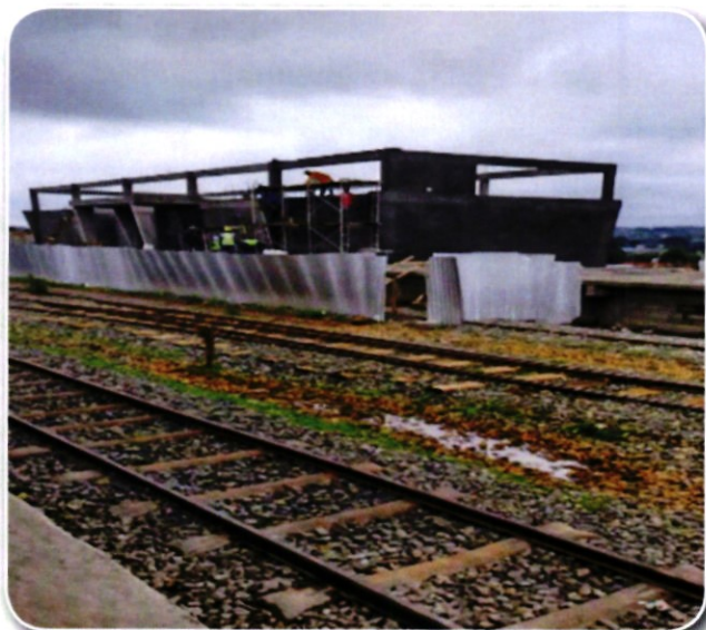
Ongoing Ol Kalou Railway Station
