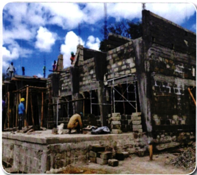
Ongoing Nyahururu Railway Station
