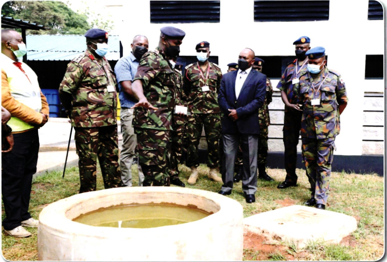
Maj Gen Peter Muteti (ACDF OPD & T) (in suit) being taken through the solid waste management and biogas system facility at the Defence Headquarters on 31 January 2022
