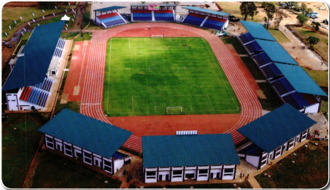
The newly constructed Ulinzi Sports Complex-Lang'ata as at 30th June 2022
