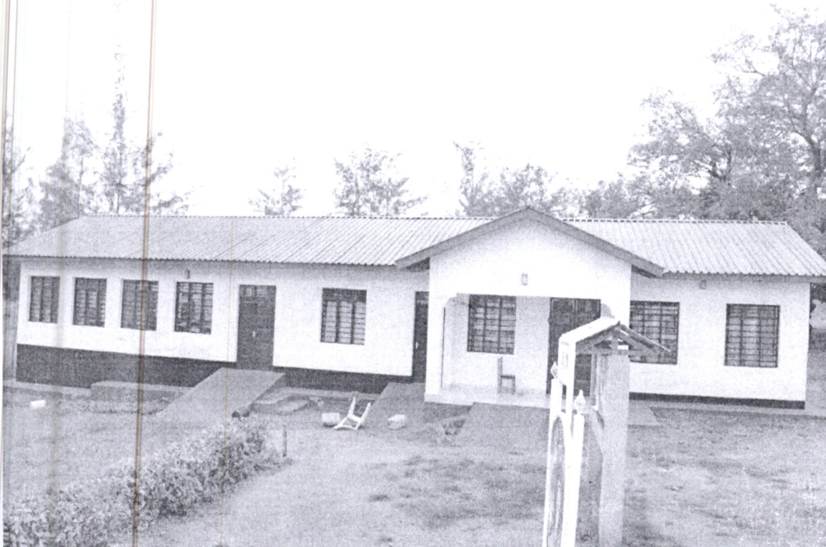
Mwenza mwenye Secondary School administration block
