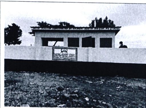
Constructed boys latrines at Korinko secondary school
