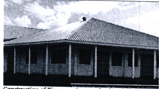
Construction of Kimana primary school multipurpose hall
