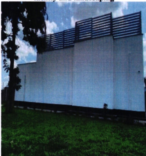
Side view of Radiotherapy Bunkers; The facility and landscaping
