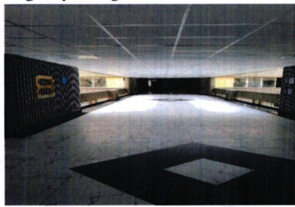
Bridge way to wings A & B
