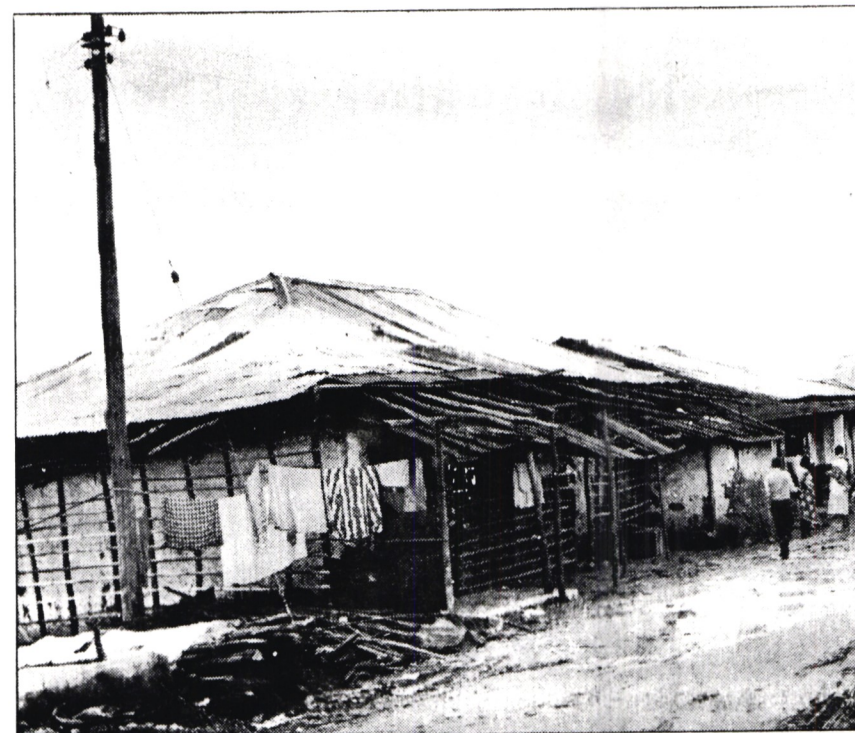
DP believes that everyone should have the chance to live in an acceptable dwelling.
