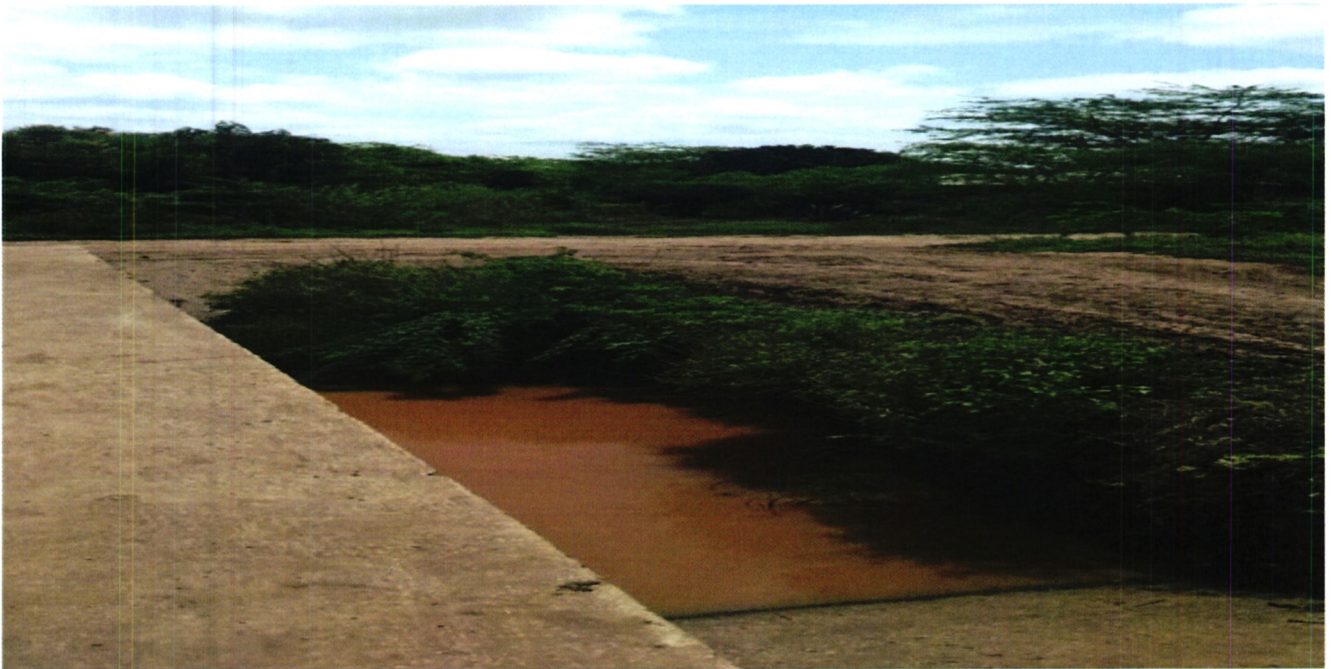
Figure 46: Repaired river brook at Tana delta Irrigation Project
