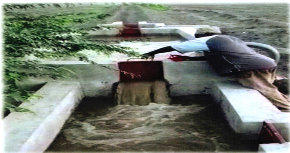
Figure 51: Water canal and distribution box at Boji
