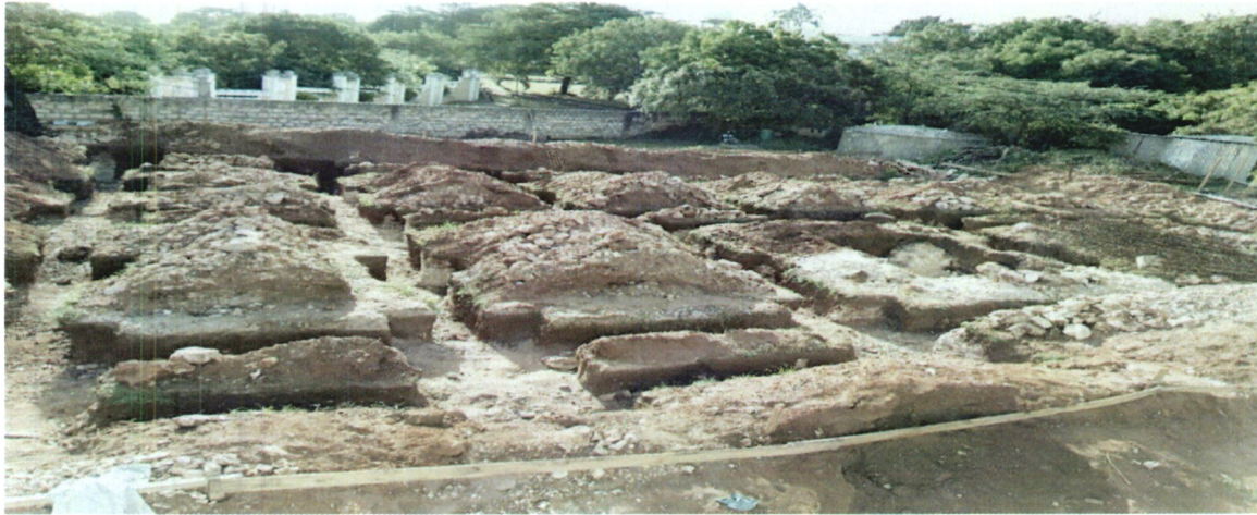
Figure 50: Foundation of the new accommodation rooms
