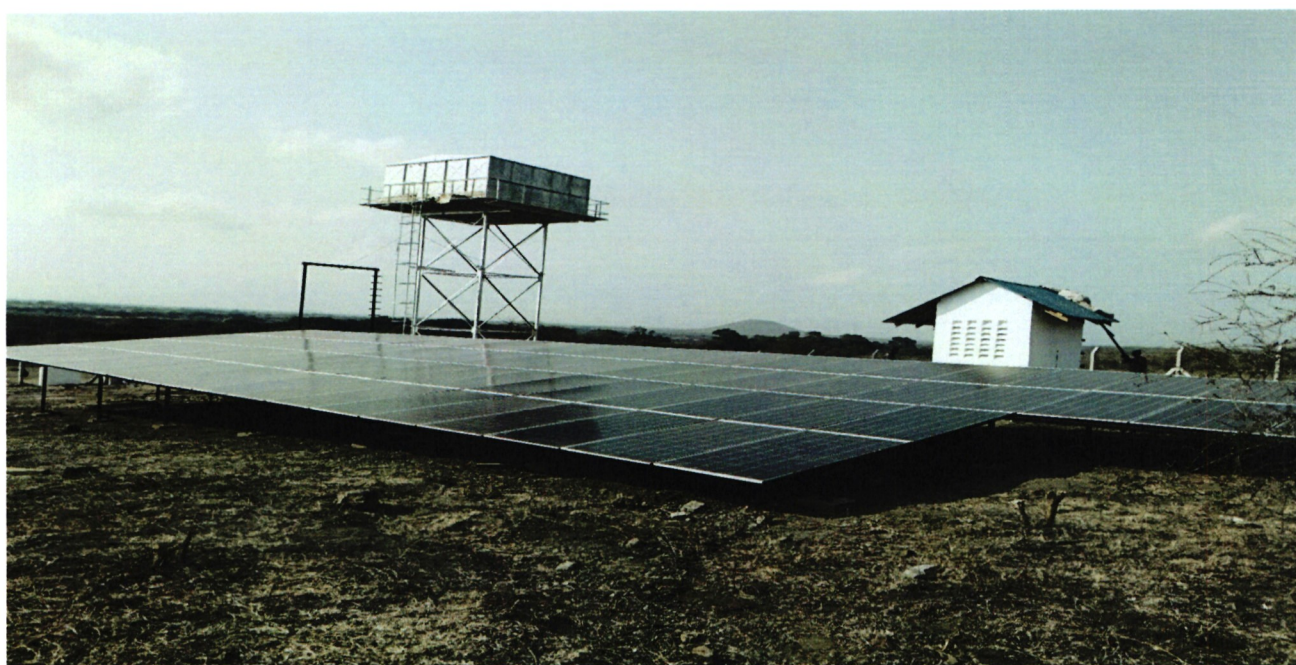
Figure 52: Solarized borehole at Nakuruto Challa
