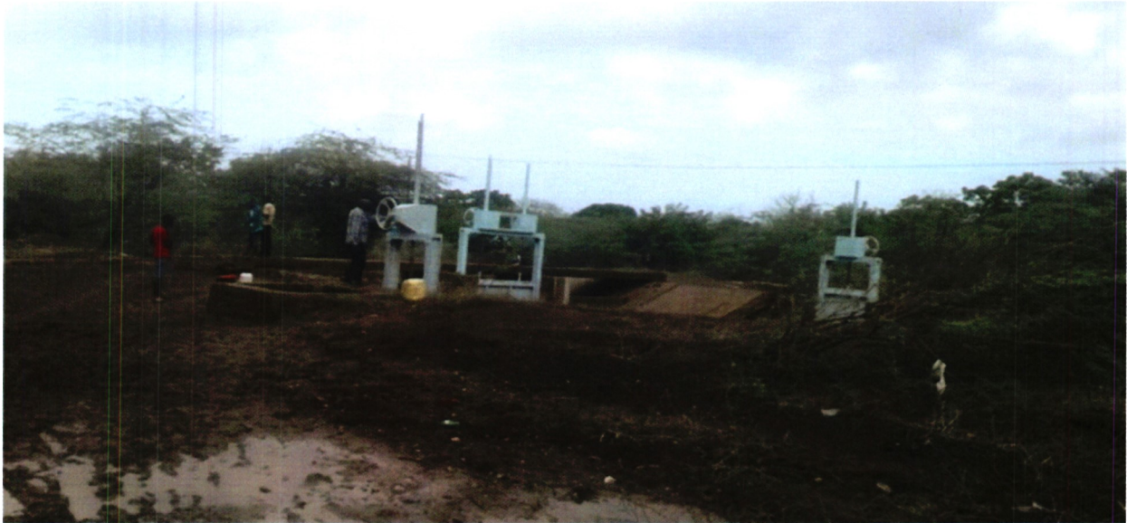
Repair of canal regulator gates at Hewani
