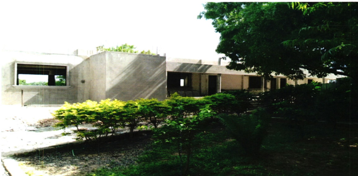
New conference facility under construction
