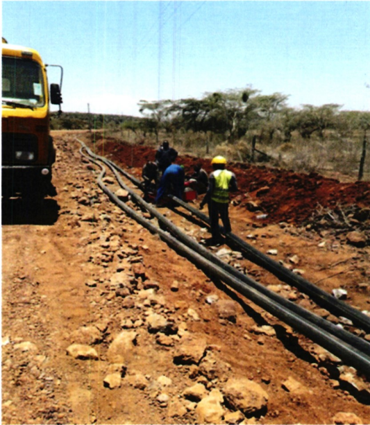
Excavation for laying of the 17 km pipel 1
