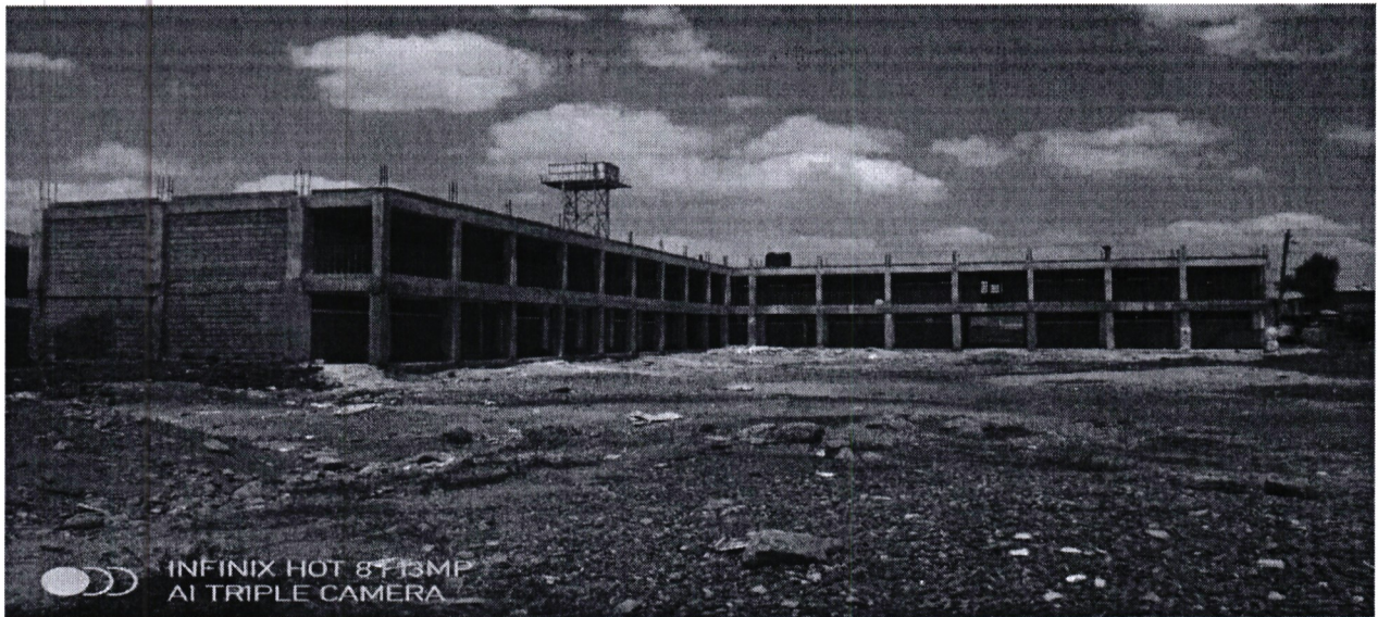
ONGOING CONSTRUCTION KWA RUBEN SECONDARY SCHOOL
