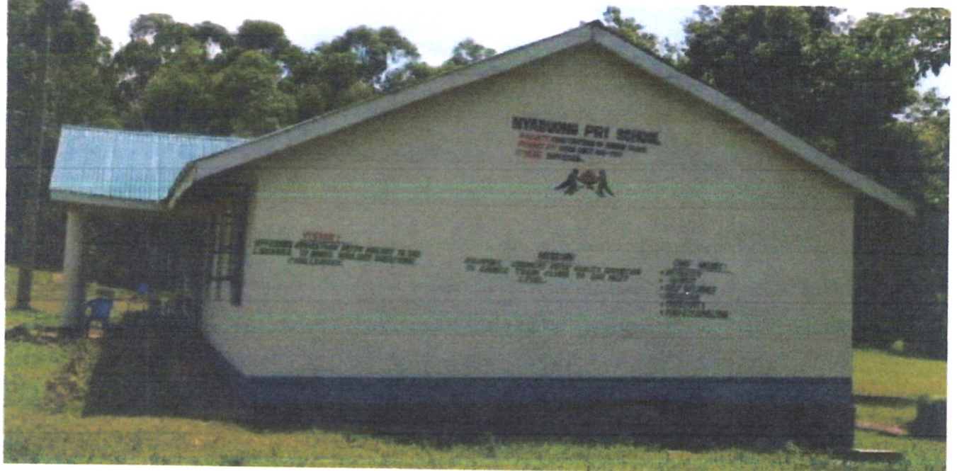
Figure 2 b Construction of the Administration block to completion.
