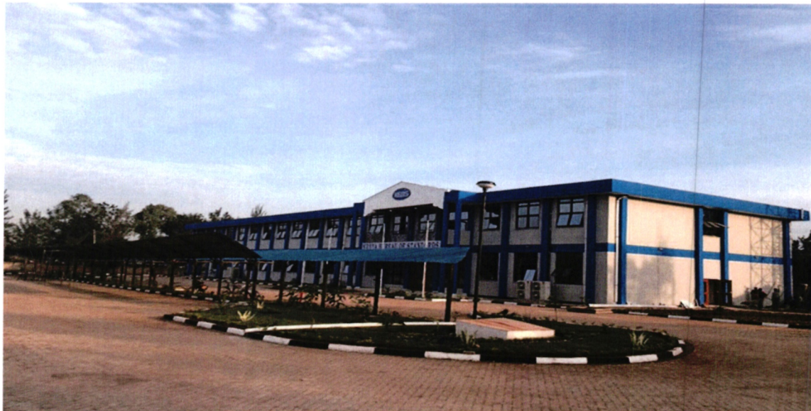
Figure 12: North Rift Regional Office and Laboratory under Construction
