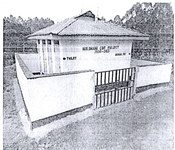
Emergency Project – Imbale Primary School
