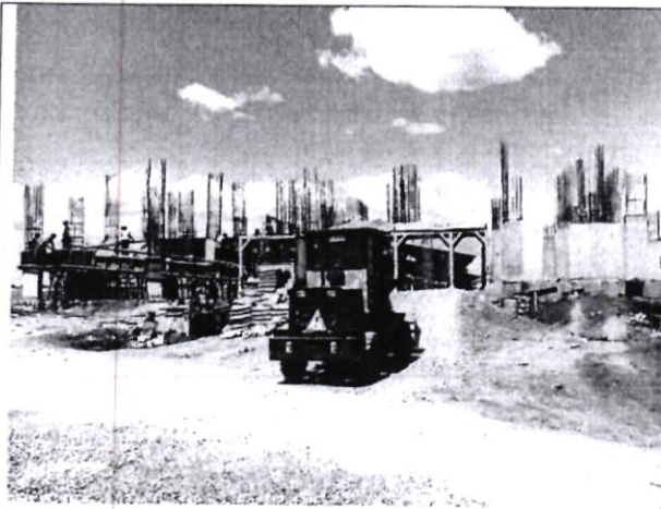
Ongoing Construction at the Tana River County Headquarters
