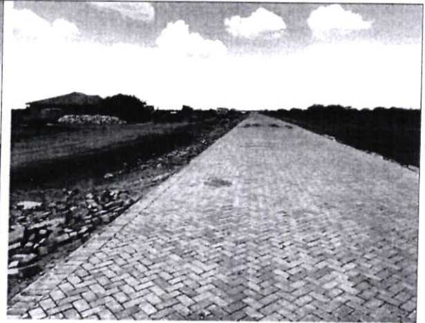
A Section of the Road to the Cluster Villages with Cabro
