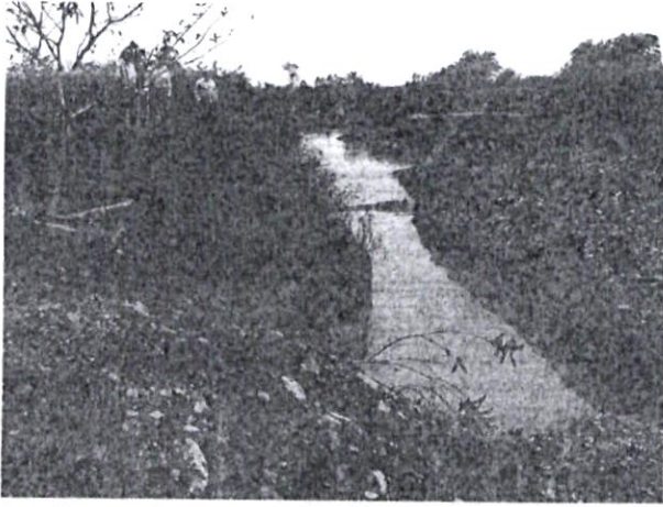
Intake works excavation for West Kenya Sugar
