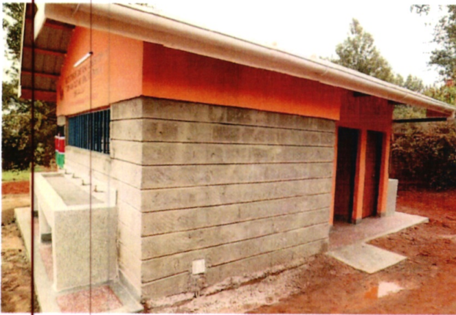
Figure 2: MUKUBU PRIMARY SCHOOL – 7 DOOR AQUA TOILET BLOCK
