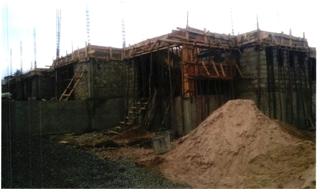
Construction of TSC Office in Bomet County
