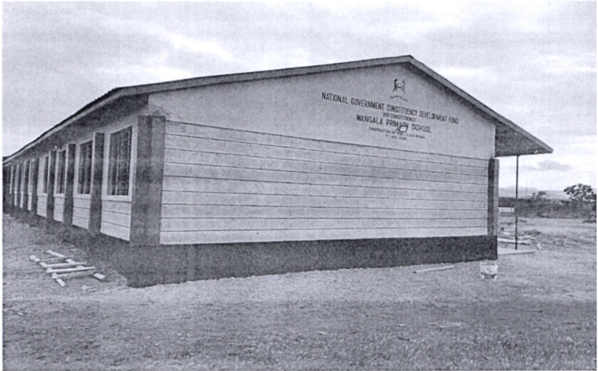
Construction to completion of 2 no. classroom at Wagalla primary school
