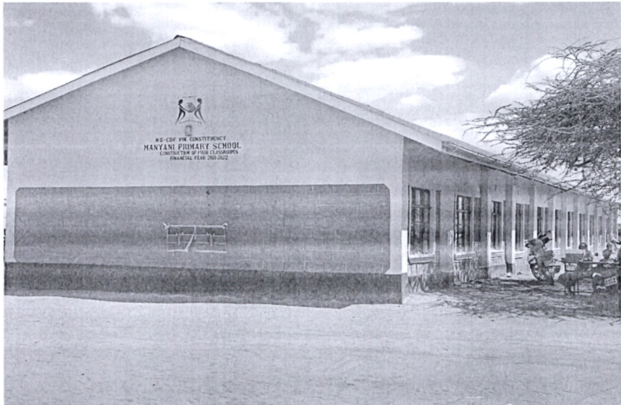
Construction to completion of 4no classroom at Manyani primary school
