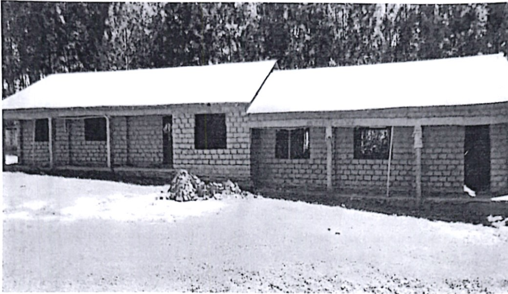
Ongoing construction of twin lab at Nakoba Friends Secondary School
