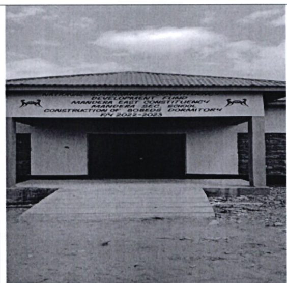
Mandera Secondary School-Construction of dormitory
