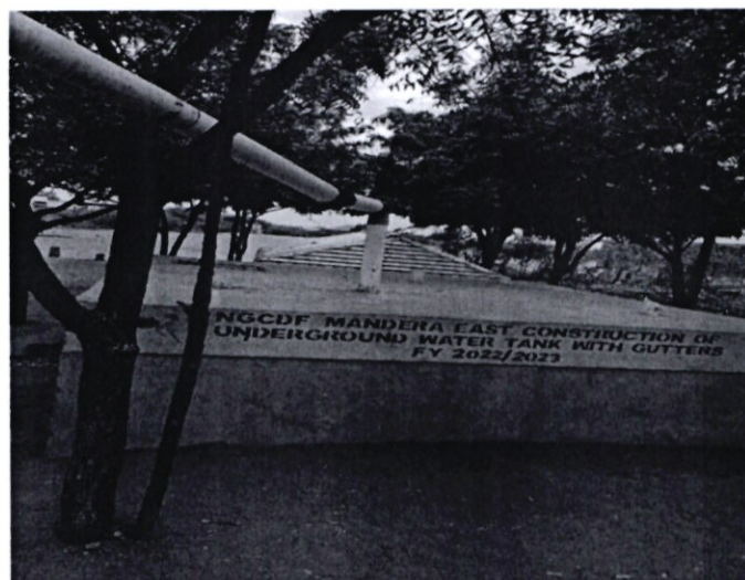
Libehiya Primary school- Construction of water tank and gutters.
