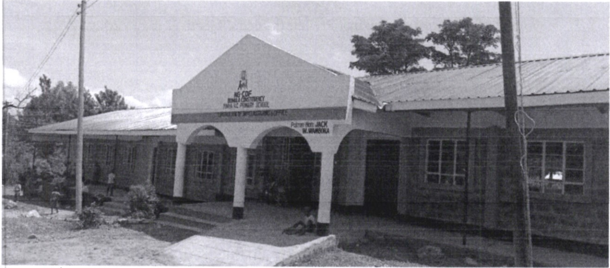
Tunya Primary School-Construction of 3 classrooms and an office
