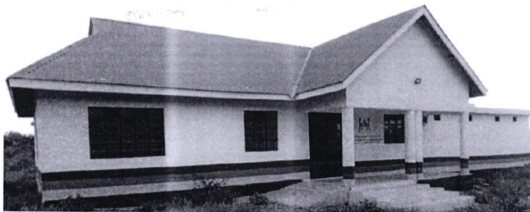
CONSTRUCTION AND COMPLETION OF POLICE POST AT NANGO POLICE STATION.
