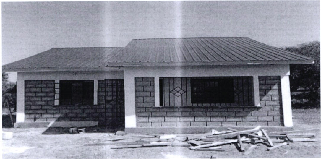
CONSTRUCTION OF STAFF HOUSE AT MARANYONA SECONDARY SCHOOL
