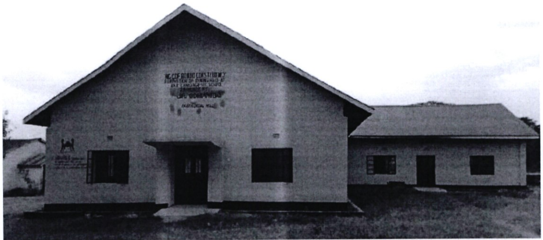
COMPLETION OF DINING HALL AT BAR-KANYANGO SECONDARY SCHOOL
