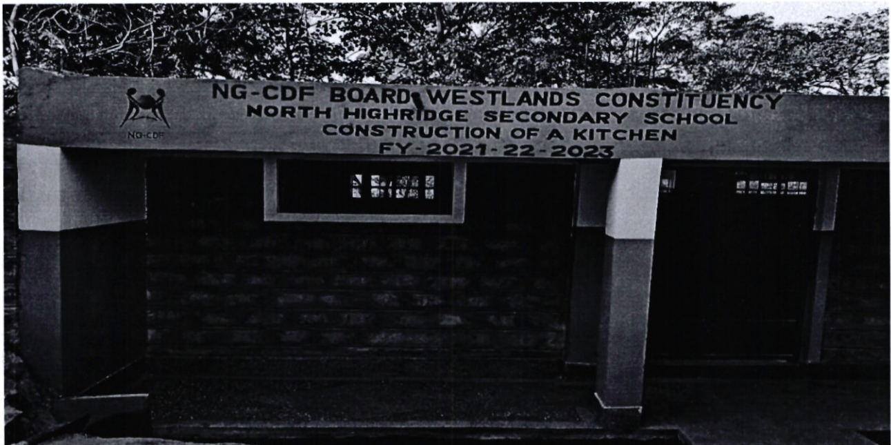
Figure 1: Construction of a Kitchen at North Highbridge Secondary School
