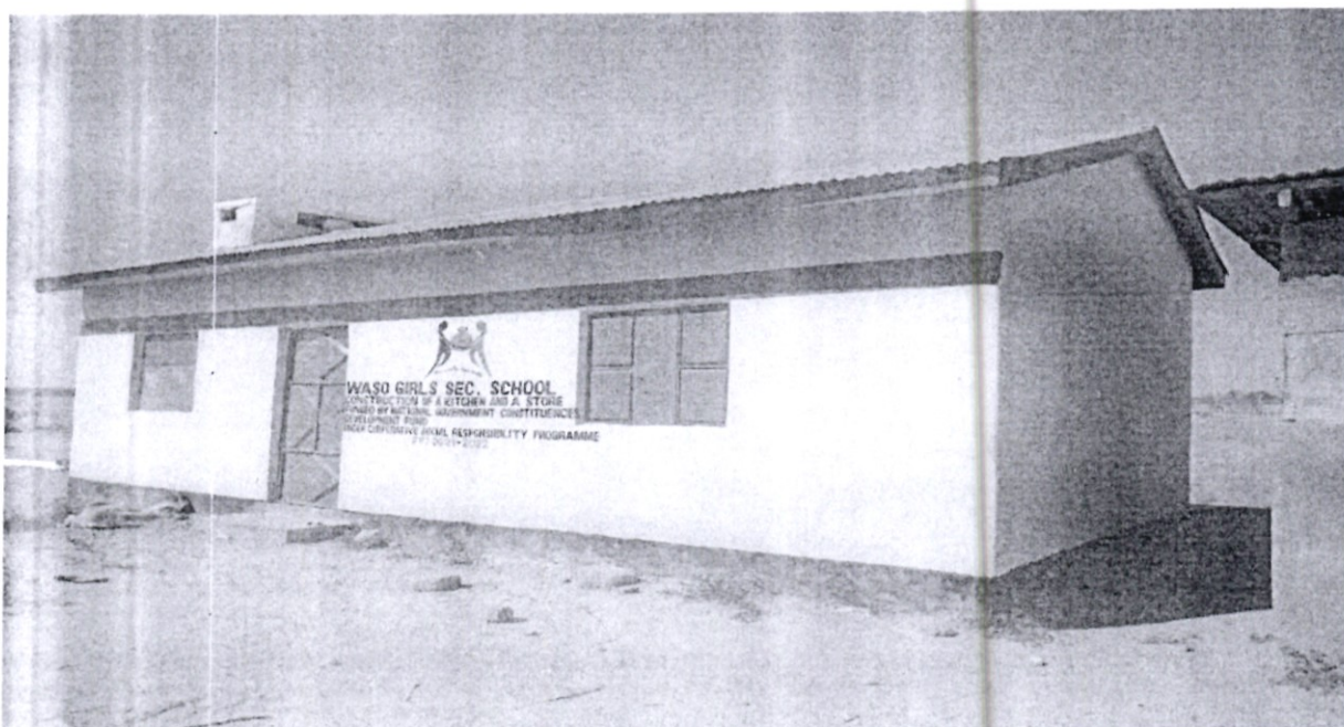
This Kitchen and store at Waso Girls Secondary School has been fully funded by Wajir West Constituency NGCDF during the FY 2021-2022 to enhance the government's policy of 100% transition by providing low cost day schools for girls.
