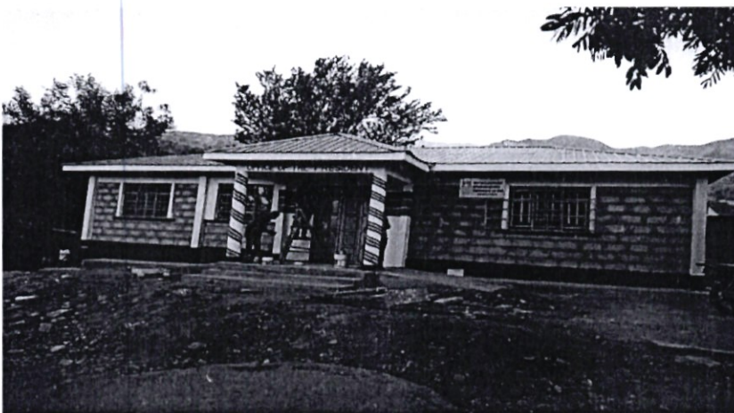
Fig. 5: Batei ACC's Office- Construction Batei ACC's office
