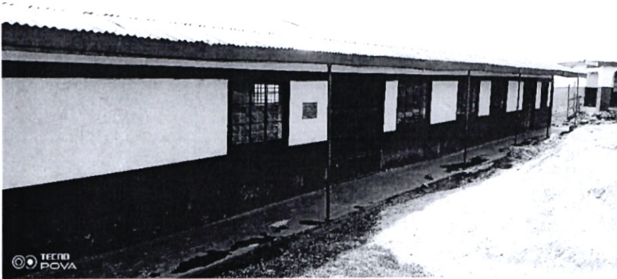
Fig. 1: Tapach primary school. Construction of Dining Hall
