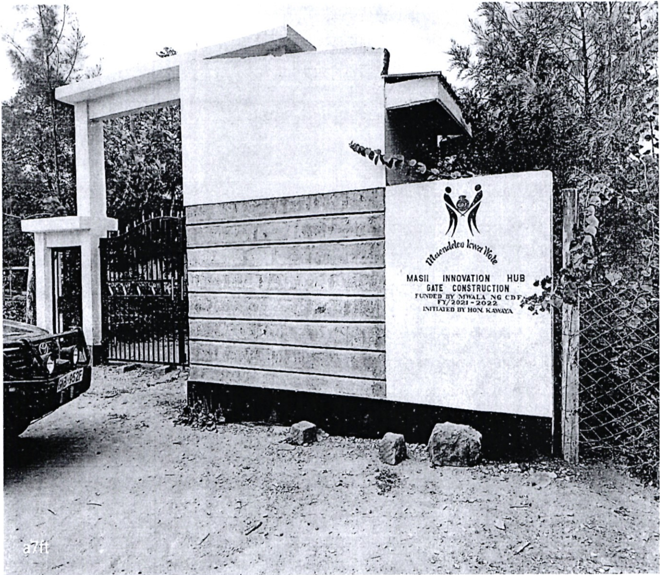
Masii innovation construction of metallic gate
