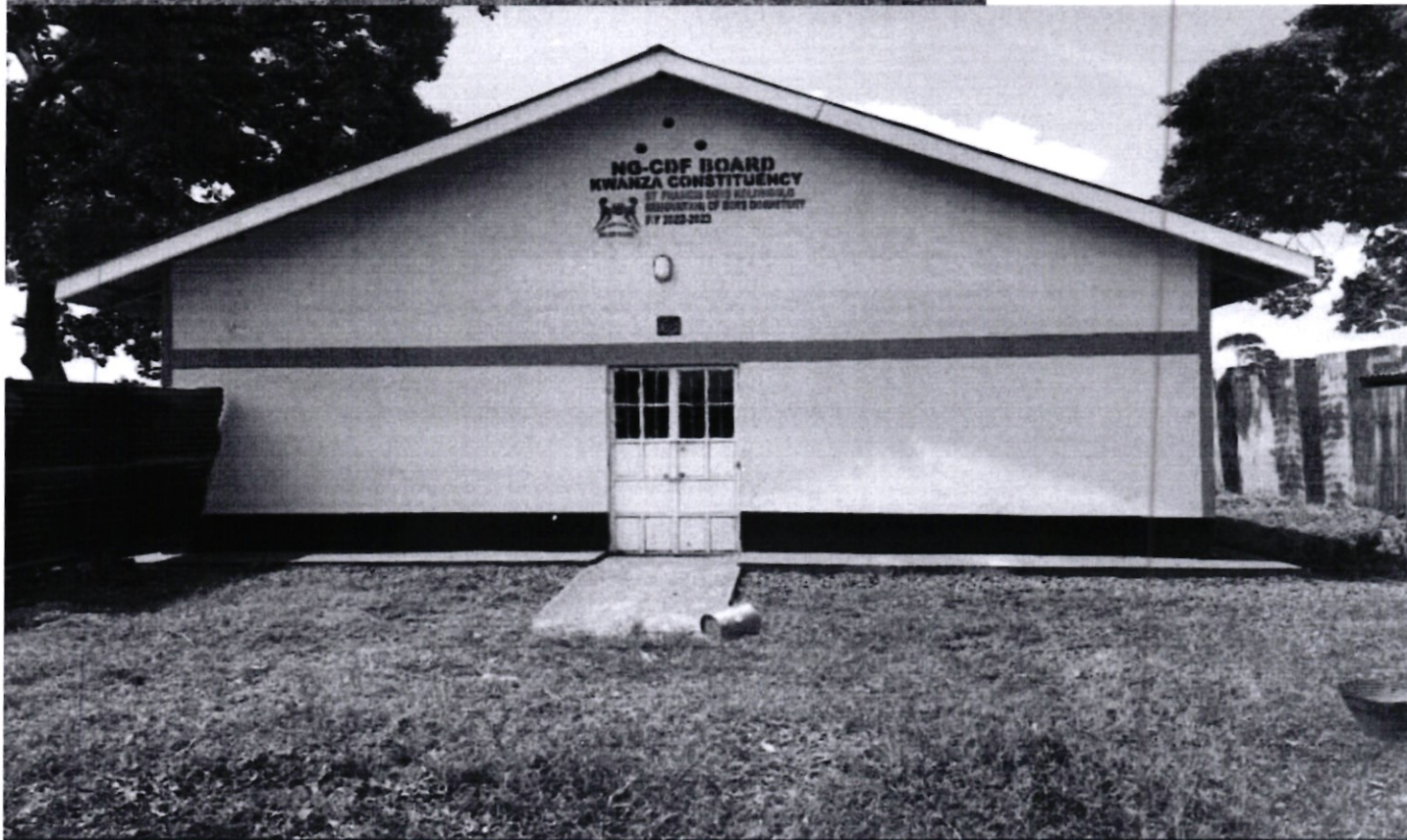
ST FRANCIS KOLONGOLO BOYS-RENOVATION OF DORMITORY-COMPLETE.
