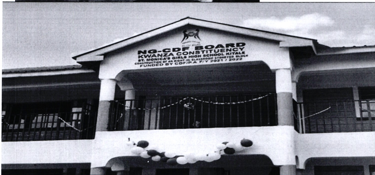
ST MONICA GIRLS HIGH SCHOOL-COMPLETION OF A STOREY BUILDING OF 8 NUMBER CLASSROOMS. -COMPLETE.
