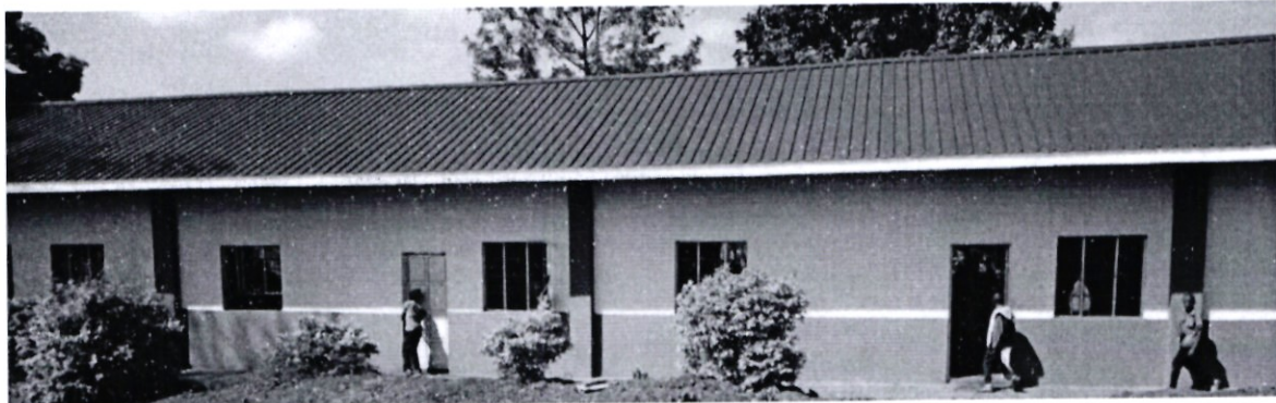
RENOVATED KIRERE PRIMARY SCHOOL CLASSES
