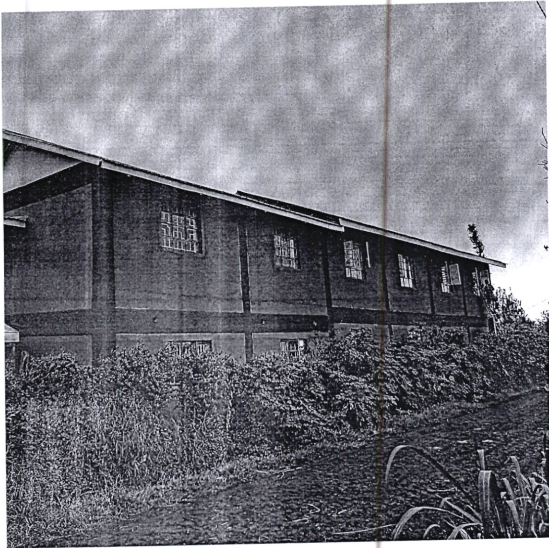
Fig 2.1 Kimaruri Primary School – Renovation of 6 No. classroom
