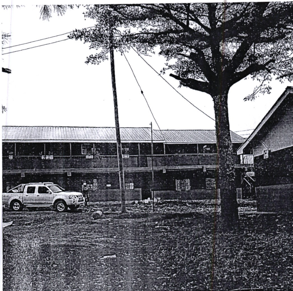
Fig 2.0 Kimaruri Primary School - Renovation of 6 No classroom
