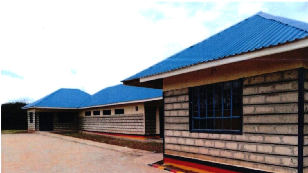
Kiirua Police Station, FY 2022/2023, Completion of Offices
