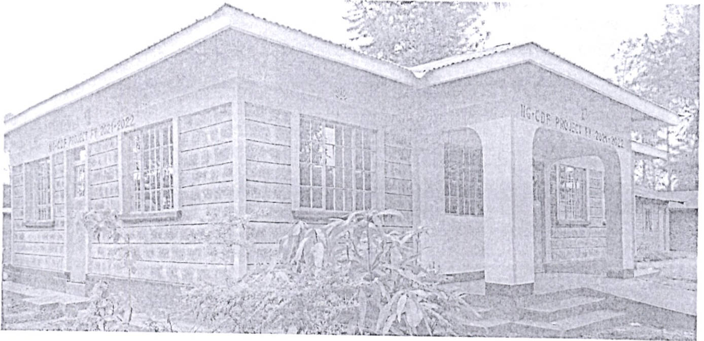
Manguliro Secondary School construction of Administration Block funded by Malava NGCDF Financial Year 2021/2022 - 2022/2023
