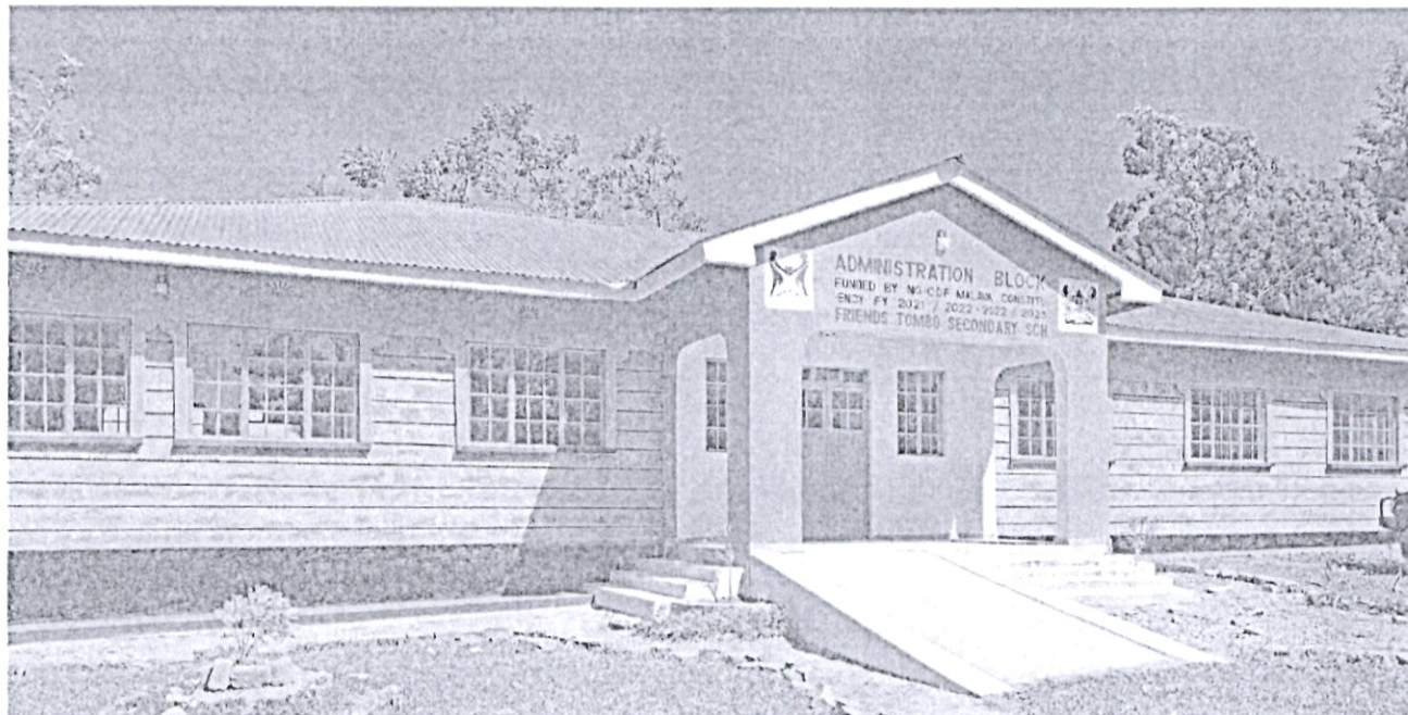
Tombo Secondary School construction of Administration Block funded by Malava NGCDF Financial Year 2022/2023
