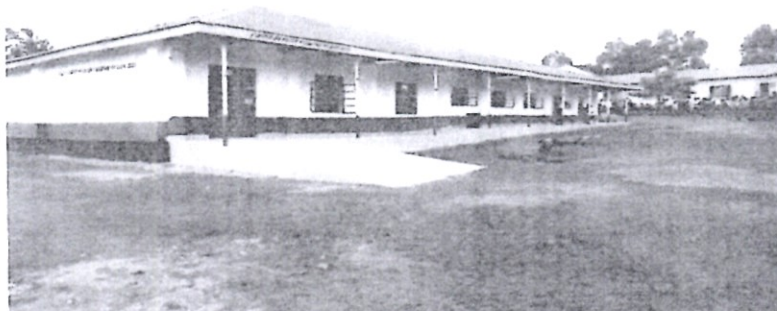
BUSAKALA SECONDARY SCHOOL – CONSTRUCTION OF LIBRARY
