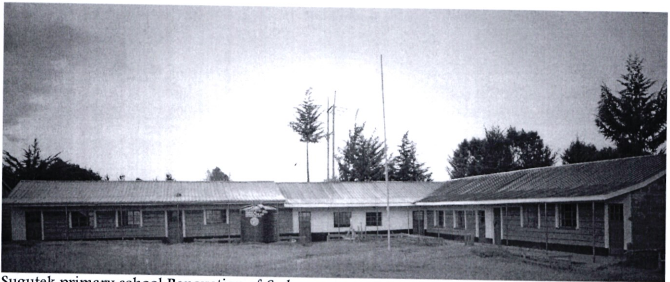
Sugutek primary school Renovation of 6 classrooms
