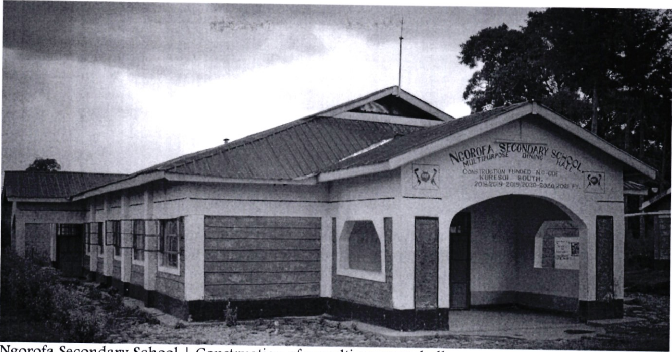
Ngorofo Secondary School | Construction of a multi-purpose hall
