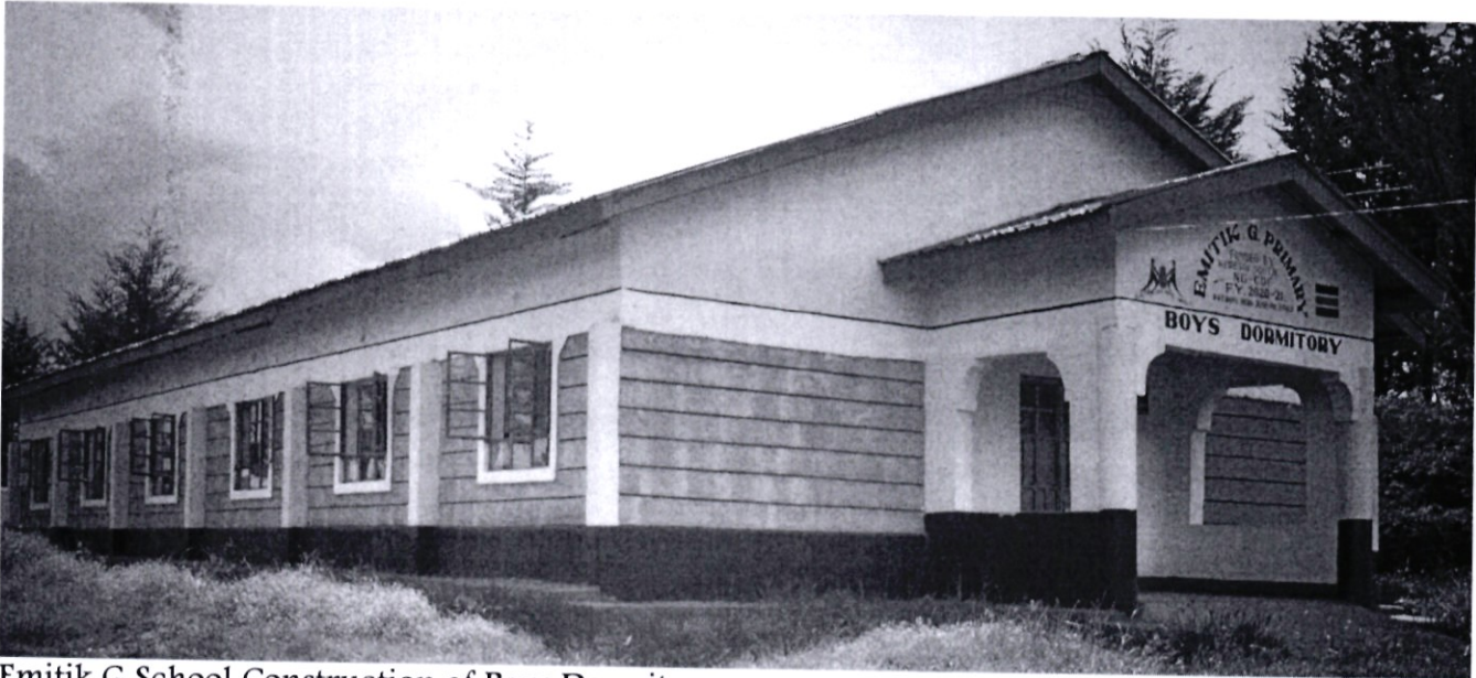
Emitik G School Construction of Boys Dormitory
