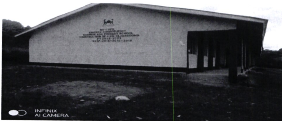
Construction to completion of 4 classroom at Sasimon ADC Primary School FY 2017-2023
