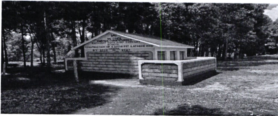
Construction to completion of 6 door latrine at Kapsabet Township Primary School FY 2022/2023
