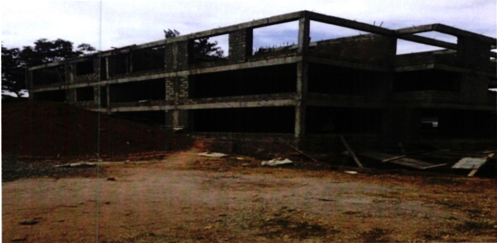
Picture 1: On-going Construction of Machakos TSC County Office
