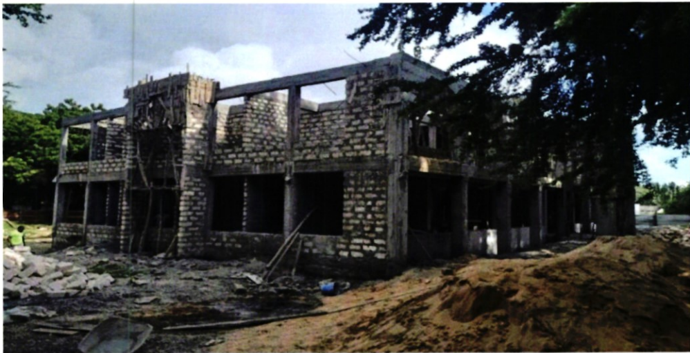
Picture 2: Ongoing Construction of Kilifi TSC County Office
