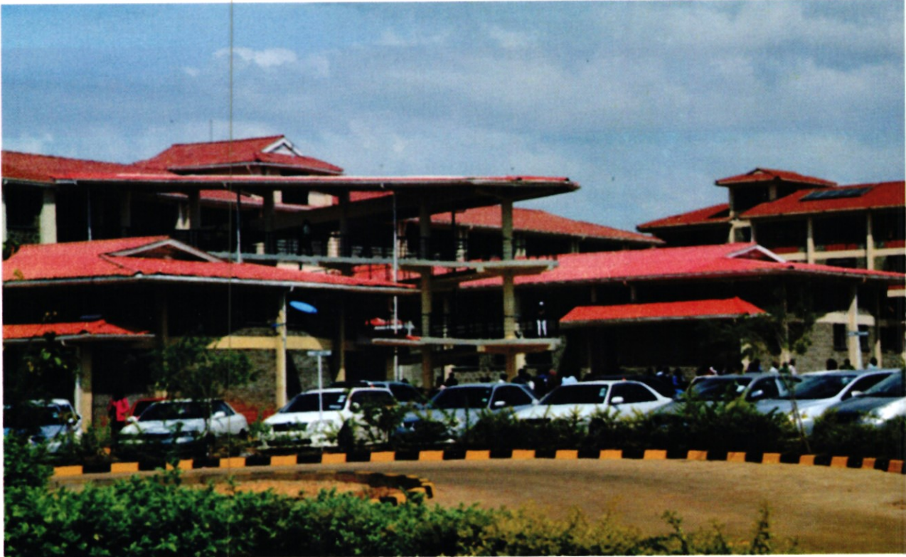
The newly constructed Phase II of the Academic Block complete with a ramp for ease of access by persons with physical challenges
