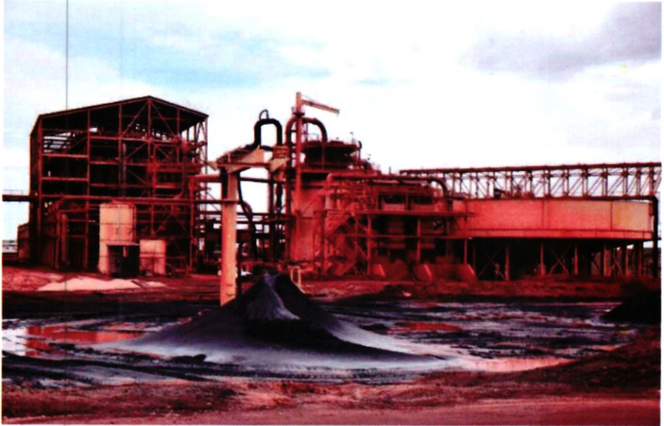
Figure 2.17 Mining Operations within Base Titanium Limited.
