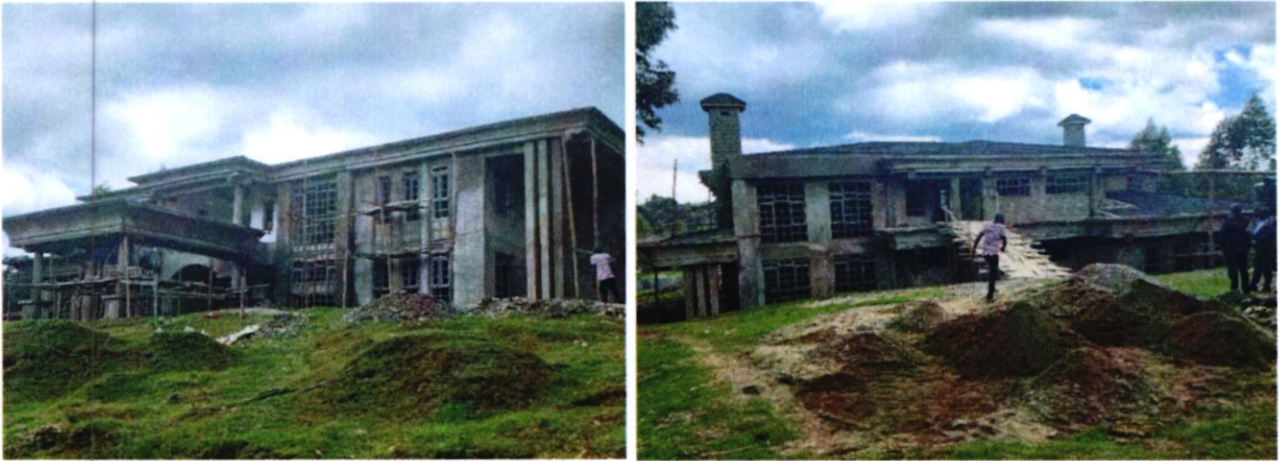
Figure 6.2: Ongoing construction of Kericho County Speaker's Residence
