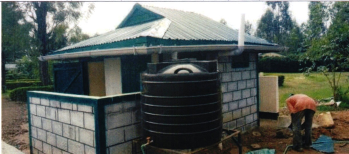
A sanitation Facility Constructed by KURA for Itando Vocational College for the deaf in Vihiga County.
