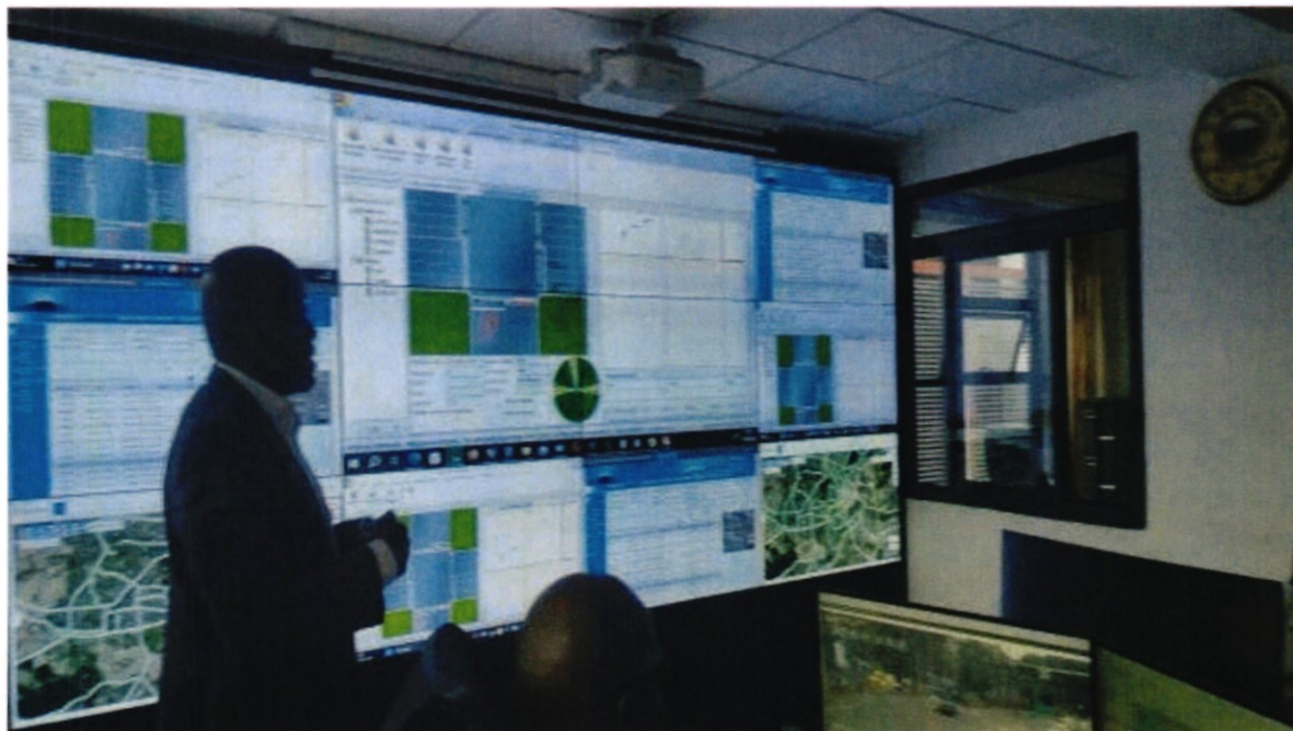
Photo Showing the Traffic Management Center where the Intelligent Traffic Management System is coordinated from.
