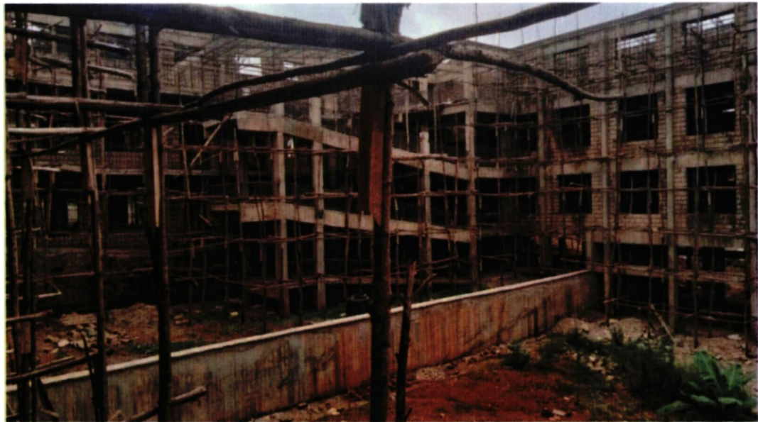
Administration Block as at 30 June 2023
