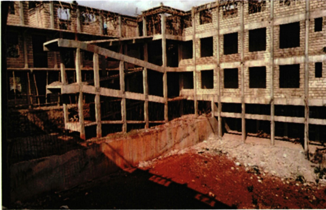
Administration Block as at 30 June 2022
