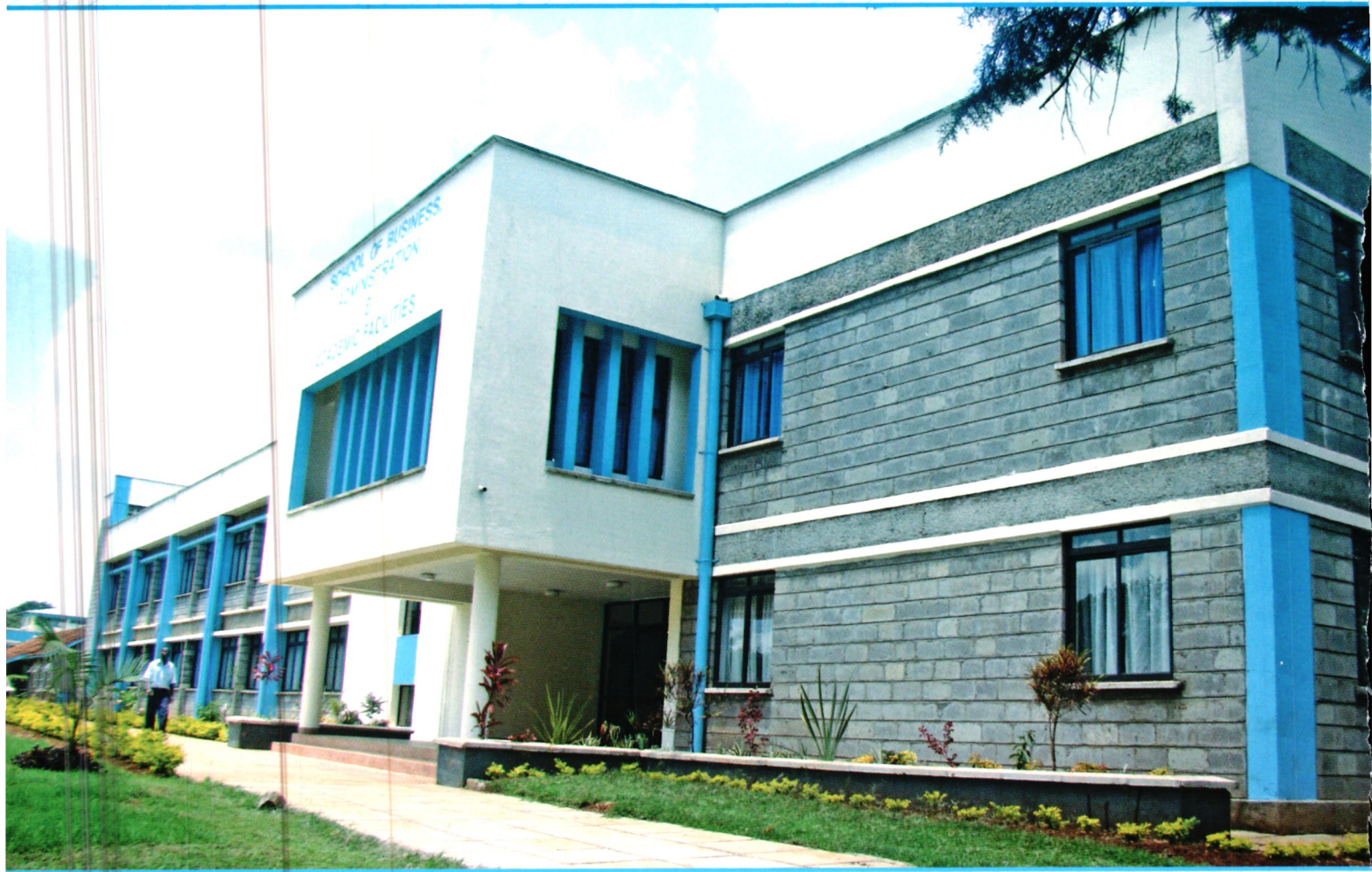
Newly completed Lower Kabete administration block
