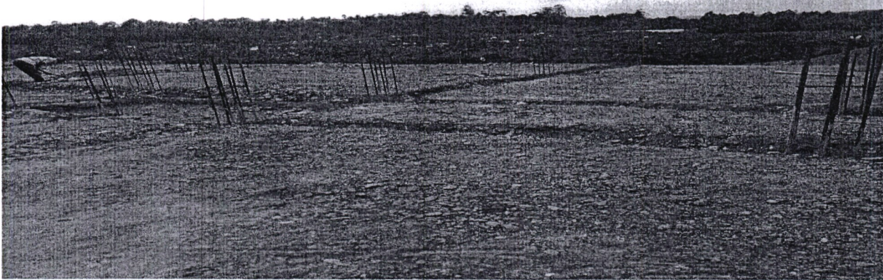
Ongoing works at Borabu Teachers Training College
