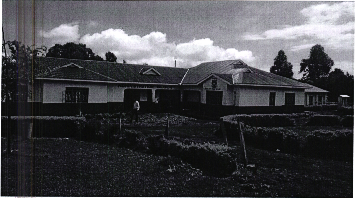
Administration block works at KIM girls on-going
