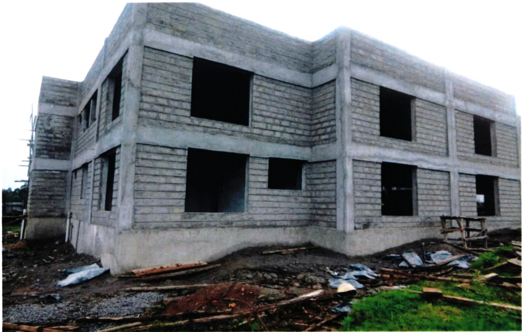
Bomet County office under construction as at June 2018
