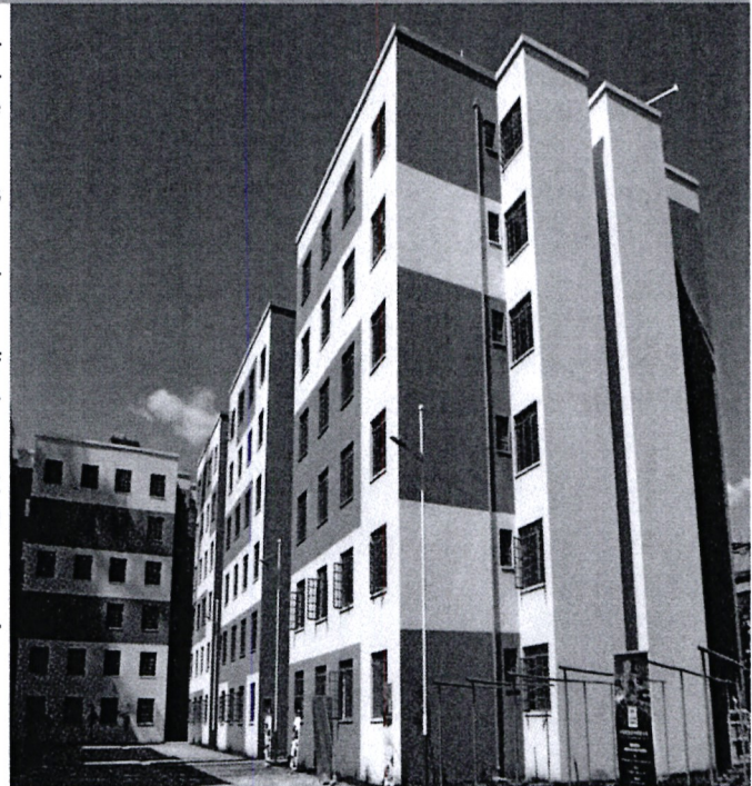
Affordable housing scheme: 228 two bedroom units at Park road completed in January 2020
