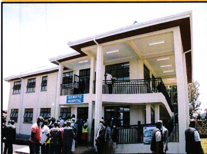
Soweto Hospital built in Kayole to bring services close to people
