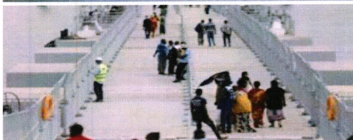
Likoni Floating Bridge has eased congestion across the Likoni Channel
