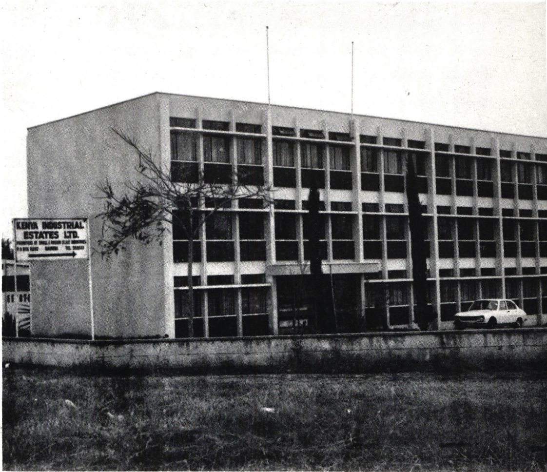
KIE Administration block.
