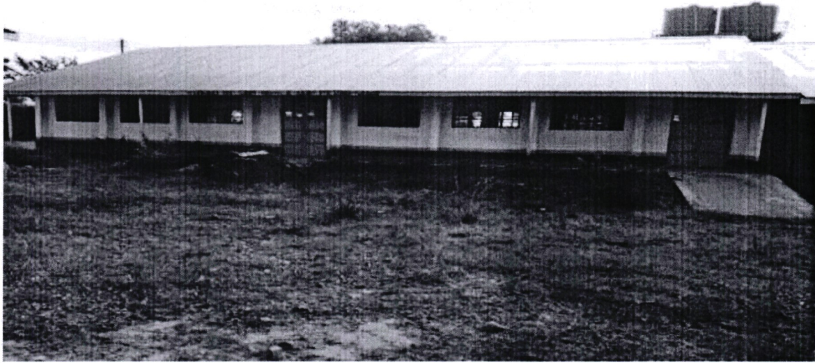
CONSTRUCTION OF 2 CLASSROOMS AT RERA KMTC FUNDED BY GEM NG-CDF
