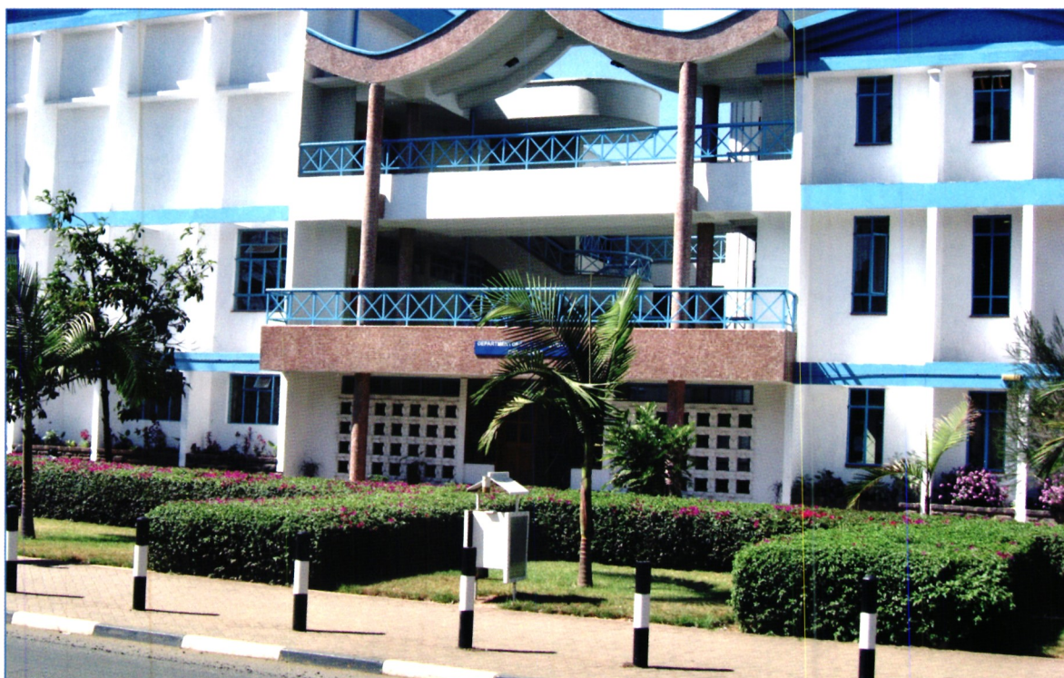
The newly refurbished civil engineering block
