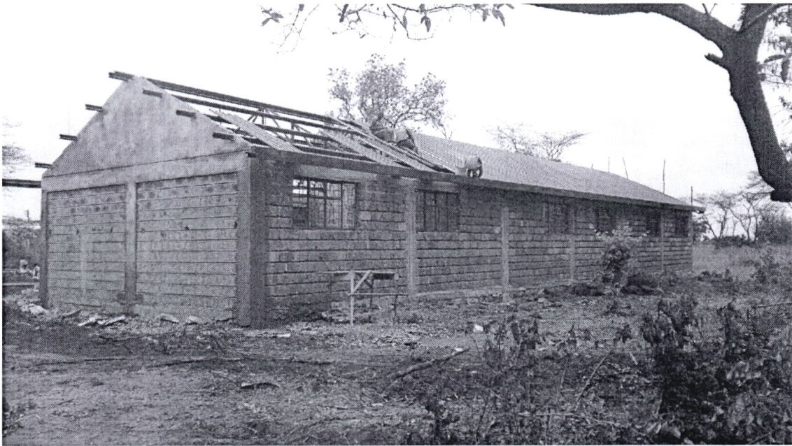
Back View of Yoghurt Factory Building
